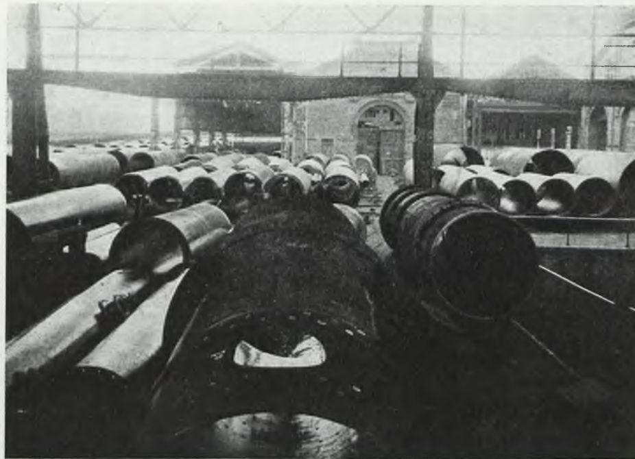
STORAGE OF WELDED PIPING MANUFACTURED BY MESSRS "FERRUM" LTD. (UP. SILESIA)
