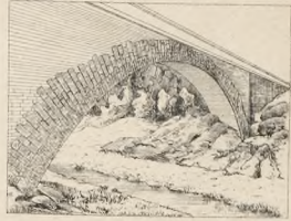
Cabin John Bridge (Aqueduct).
