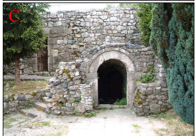
Fig. 2. Photographs from the fortress in Banja Luka. General throw (A), a fragment of the walls with visible ultrabasic rocks (B), one of the bastions and a portal to the underground corridors with visible rocks alkaline (C).
