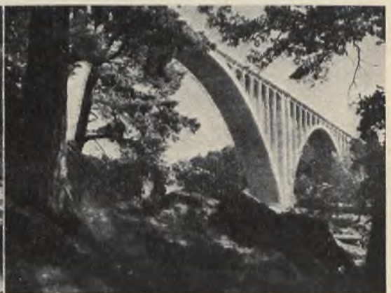
Stockholm, Skurusund. One of the largest ferro-concrete bridges in Europe.
