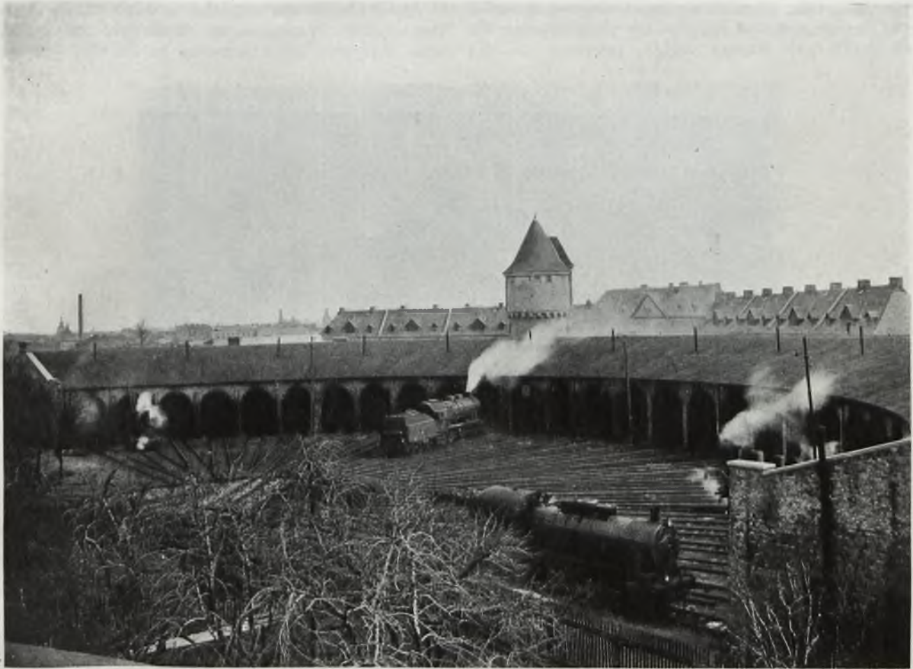
THE SAME SHED RECENTLY COMPLETED
