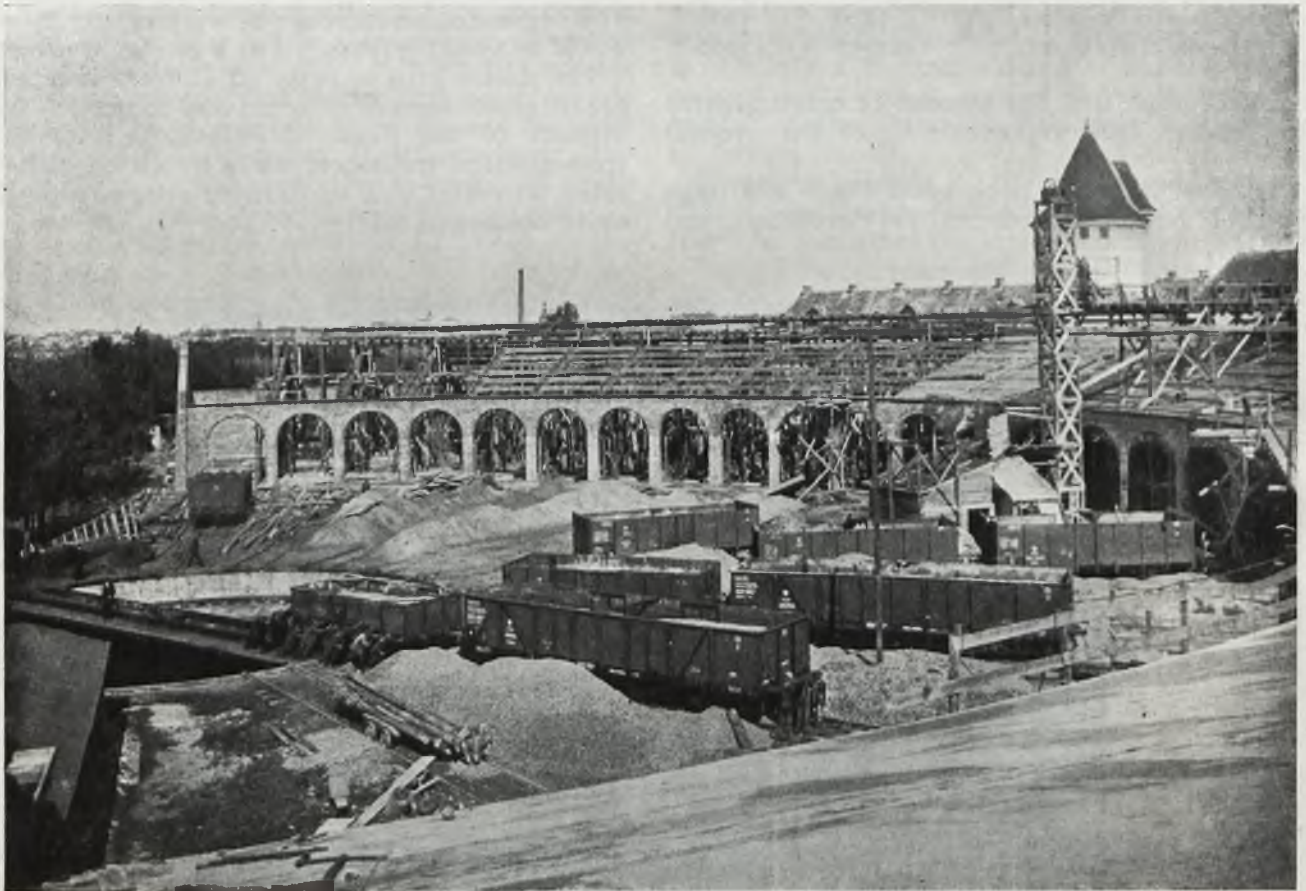
LOCOMOTIVE SHED UNDER CONSTRUCTION NEAR WARSAW
