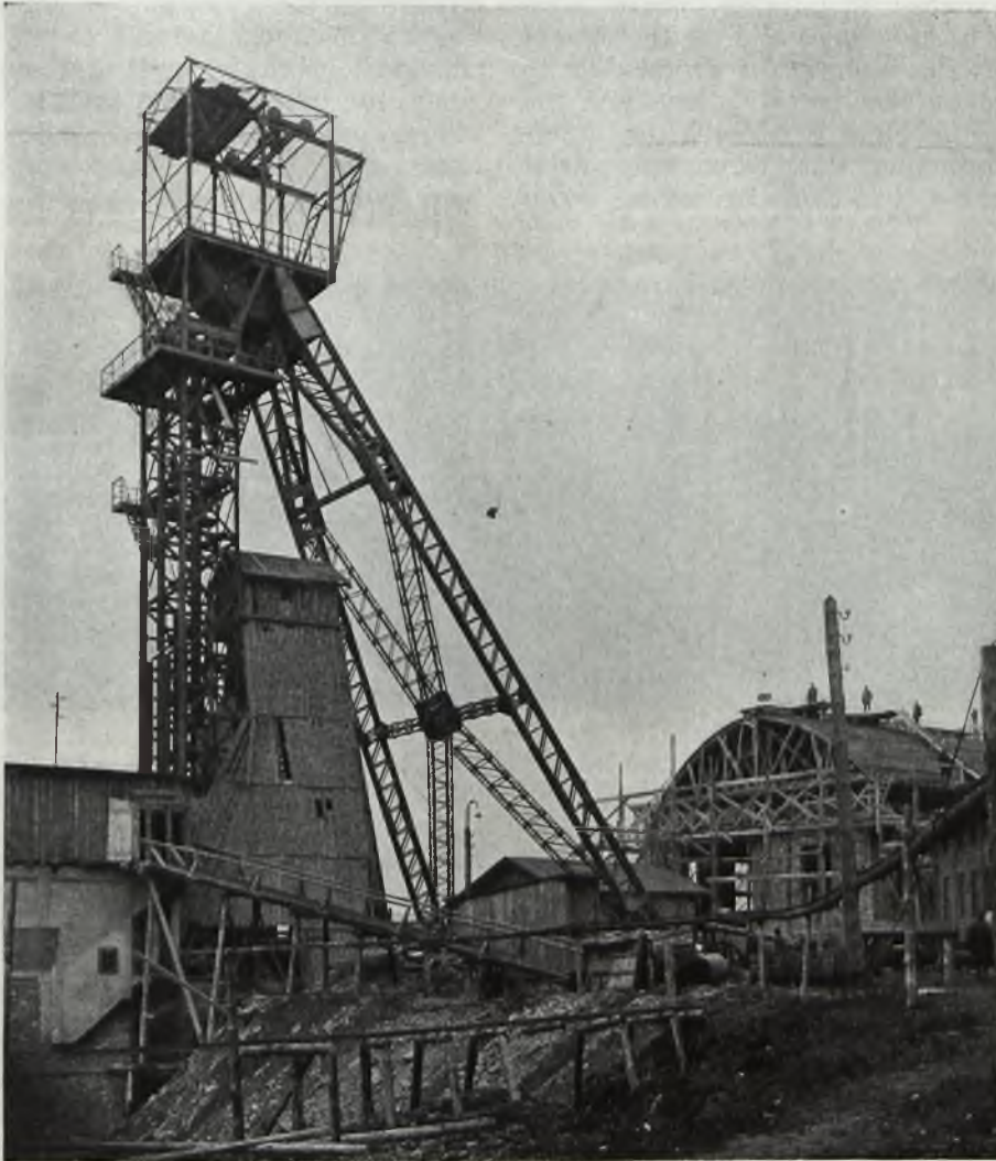
SINKING OF A NEW COAL PIT
