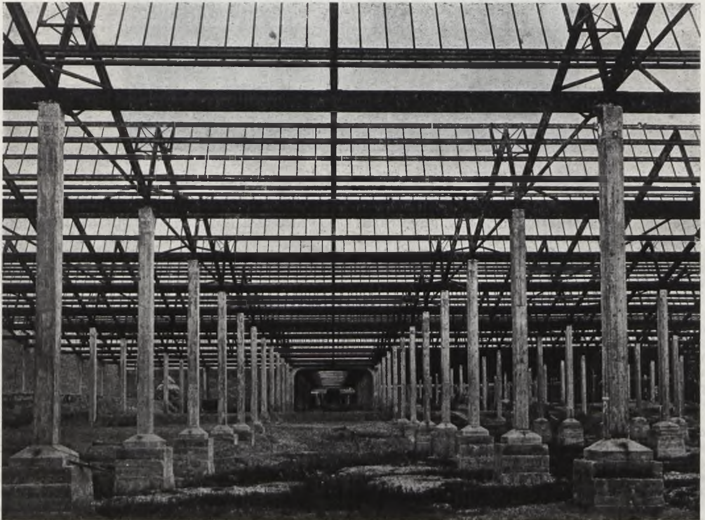
ARTIFICIAL SILK PLANT, UNDER CONSTRUCTION
