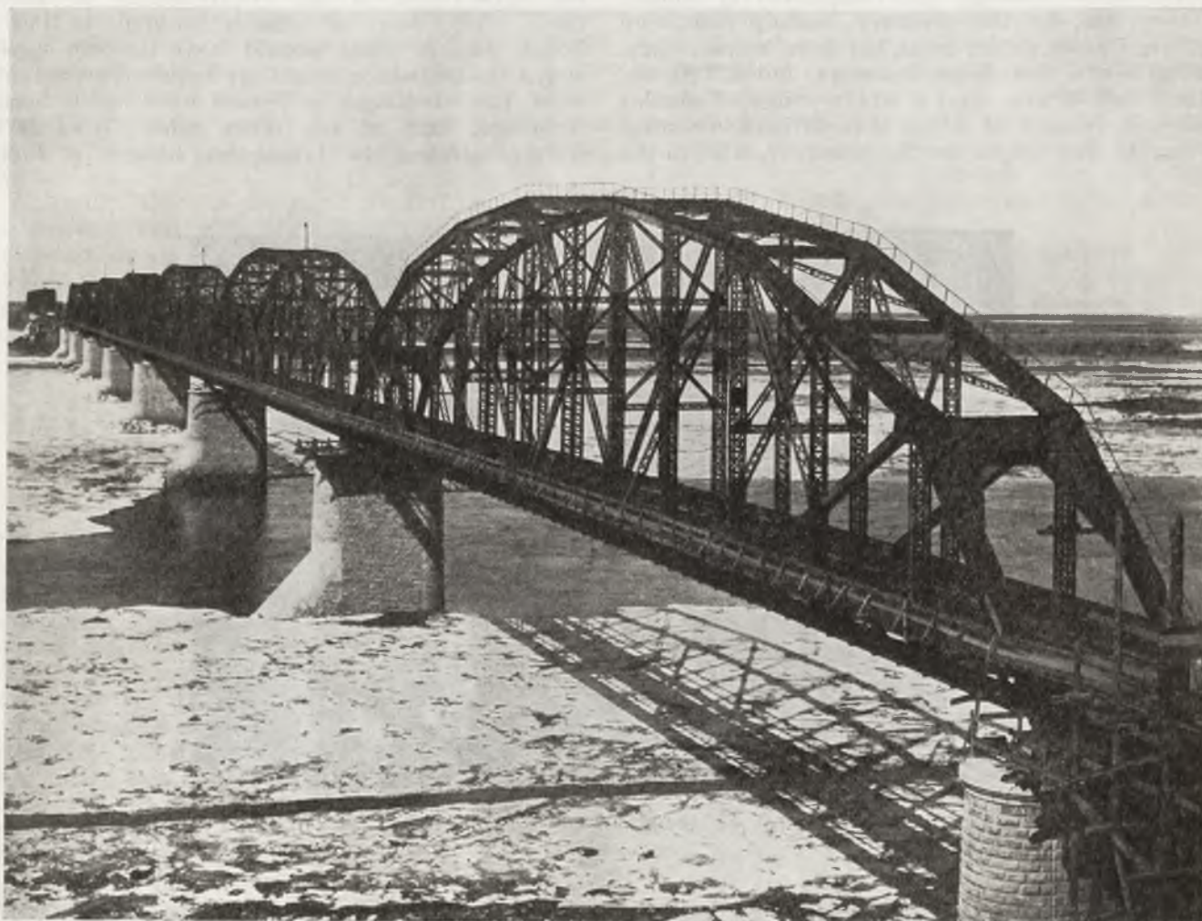
THE LONGEST BRIDGE ON THE OLD CONTINENT, CROSSING THE RIVER AMUR NEAR CHABAROWSK (SIBERIA), 2,598 M. LONG, CONSTRUCTED BY MESSRS "K. RUDZKI I S-KA", WARSAW, IN 1904/6
