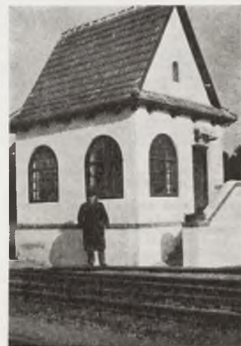
A TYPICAL SIGNAL BOX ON THE POLISH STATE RAILWAYS
