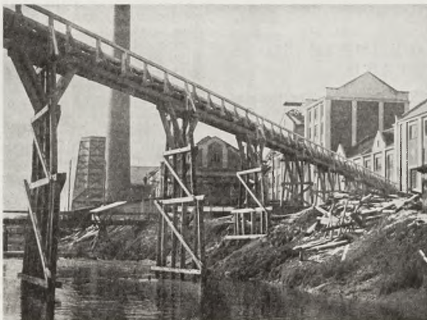
A PORTION OF THE NEWLY ERECTED POTASSIUM SALT CONCENTRATING WORKS AT KAŁUSZ (PHOT. S. PLATER)
