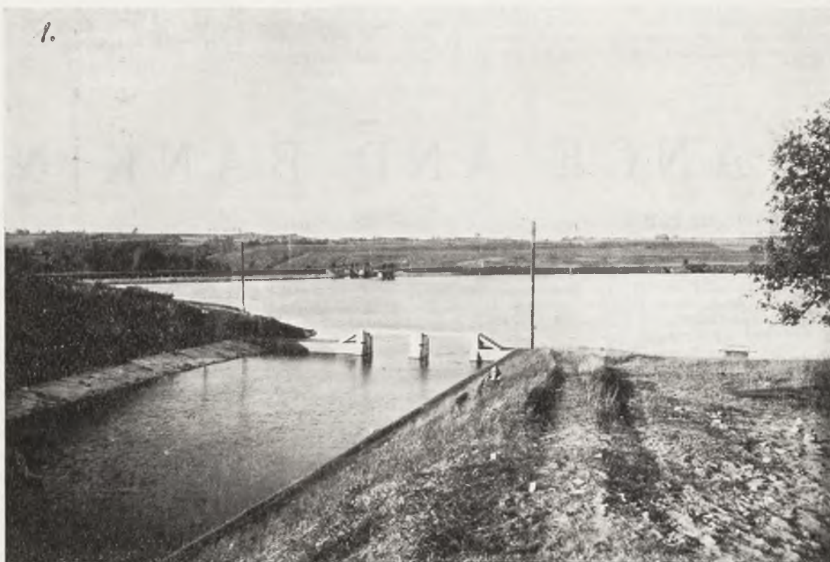
WATER SUPPLY OF THE ELECTRICAL POWER STATION AT GRODEK (POMERANIA)
