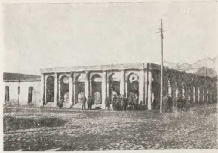
21. THE SOCHACZEW MUNICIPAL SLAUGHTER HOUSE AFTER DESTRUCTION BY FIRE
