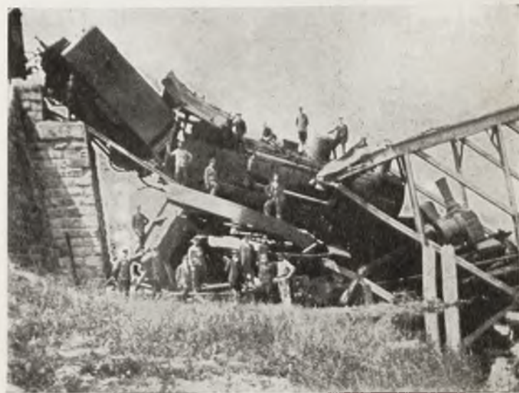
18. — A PORTION OF A BRIDGE DESTROYED BY THE AUSTRIANS
