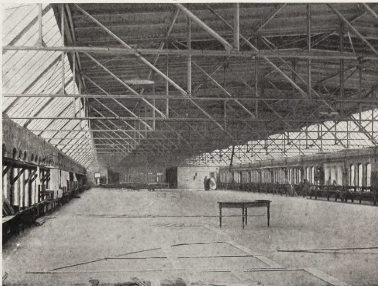
DRAWING OFFICE AT THE "INTERNATIONAL SHIPBUILDING AND ENGINEERING CO. LTD.", DANZIG, WHERE THE HUGE DESIGNS ARE PREPARED IN NATURAL SIZES
