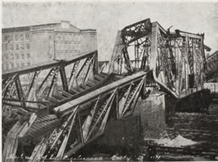
A BRIDGE NEAR CZĘSTOCHOWA DESTROYED DURING THE GREAT WAR
