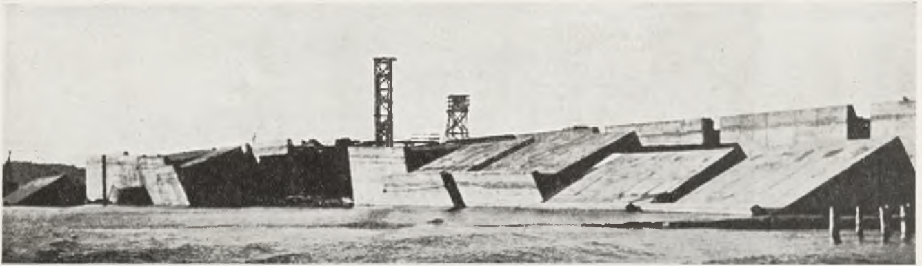
SINKING OF CONCRETE AND WOOD CAISSONS AT THE PORT OF GDYNIA
