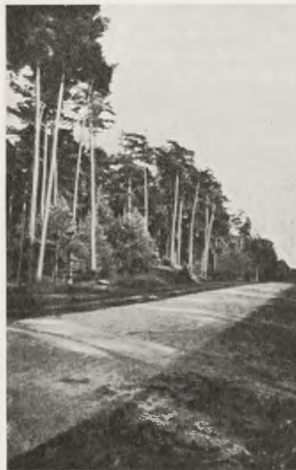
A NEWLY CONSTRUCTED FOREST HIGHWAY
