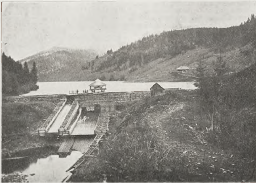
A WATER BASIN IN THE GRÓDEK ELECTRICAL POWER STATION, POMERANIA
