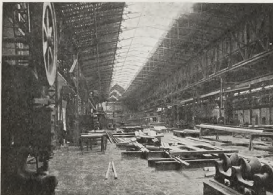
INTERIOR OF ONE OF THE SHOPS AT A BOILER AND IRON CONSTRUCTION WORKS (PHOT. S. PLATER)
