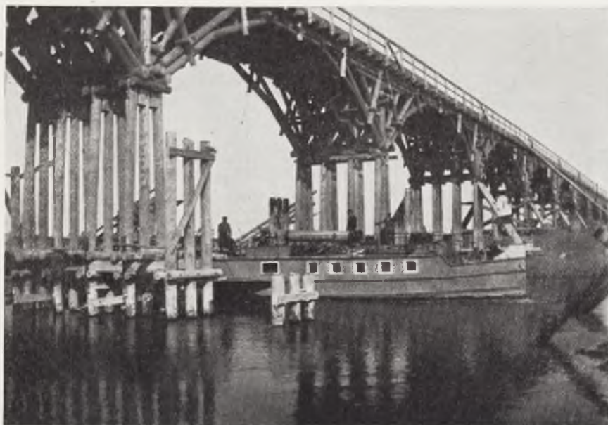
THE CONSTRUCTION OF A PROVISIONAL TIMBER BRIDGE OVER THE RIVER BUG
