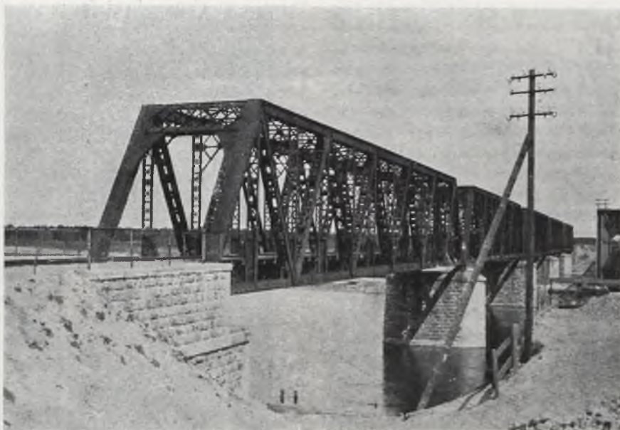
RAILWAY BRIDGE OVER THE BUG RIVER NEAR MALKINIA (PHOT. S. PLATER)
