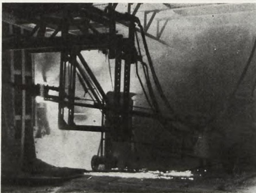
CARBIDE OVEN AT THE STATE NITROGEN COMPOUNDS FACTORY AT CHORZÓW (PHOT. S. PLATER)
