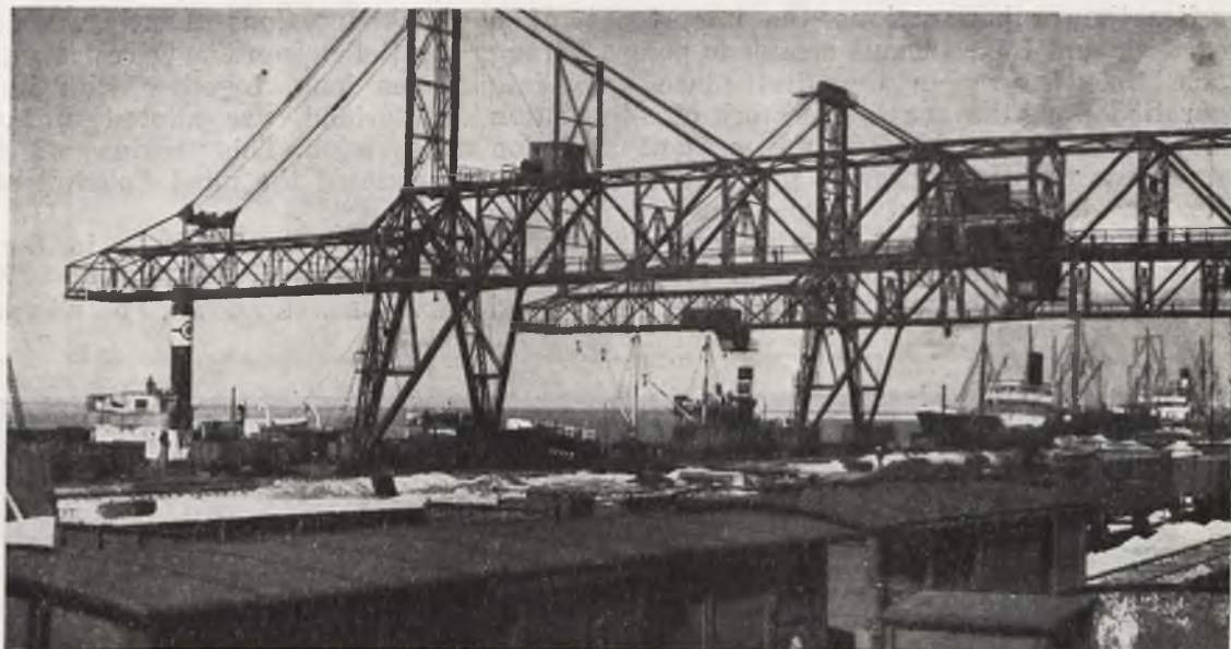
ONE OF THE CRANES AT THE
