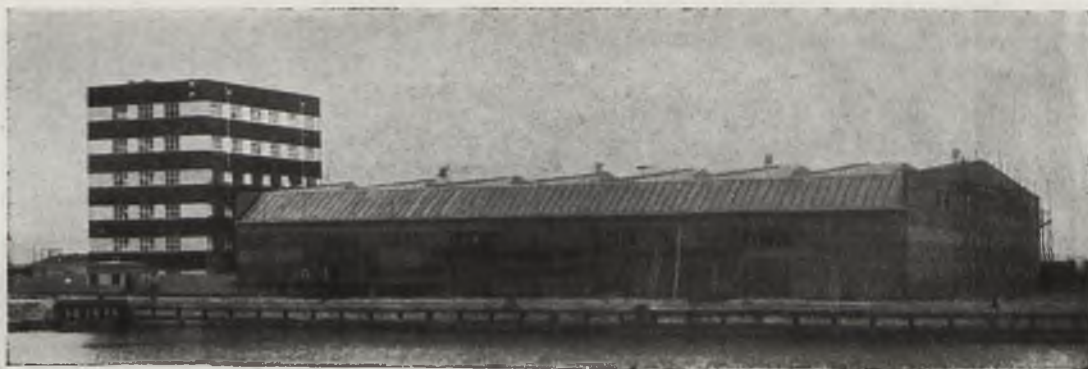
RICE HUSKING PLANT, GDYNIA (PHOT. S. PLATER)
