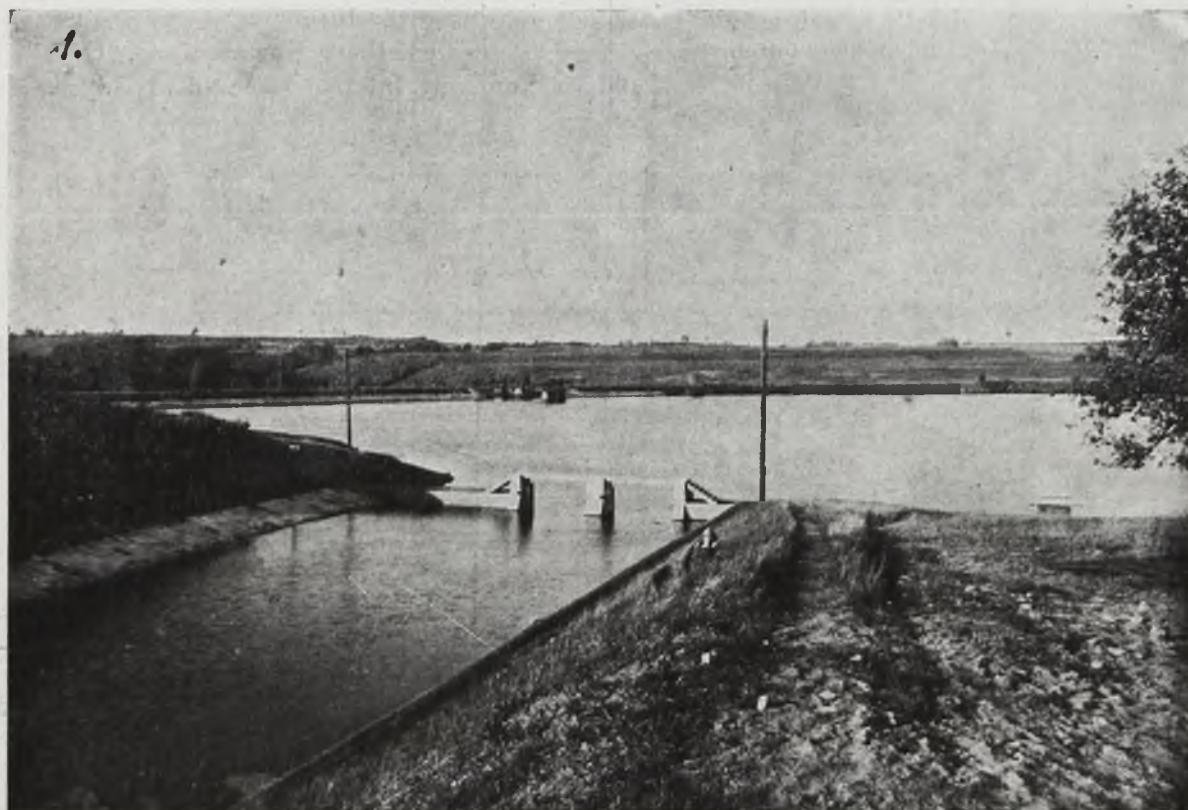
WATER SUPPLY OF THE ELECTRICAL POWER STATION AT GRÓDEK, POMERANIA
