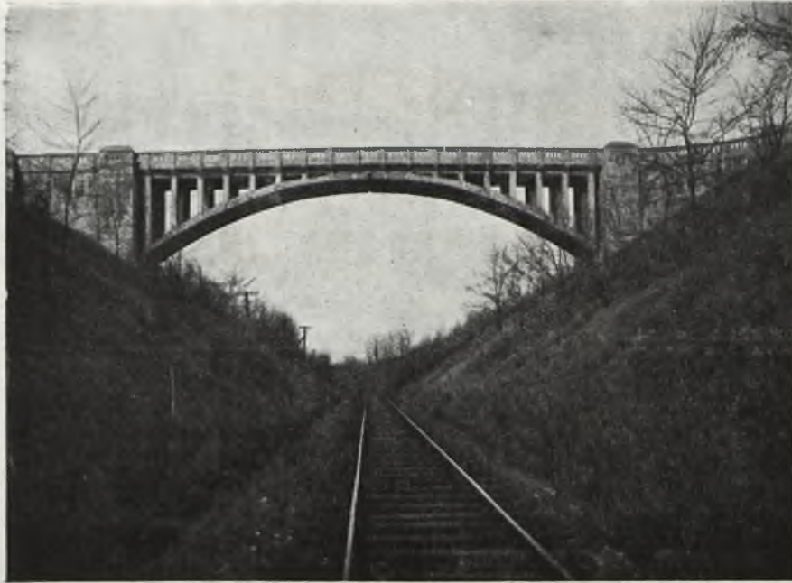
A SECTION OF THE NEWLY CONSTRUCTED JASTRZĘBIE—ZDRÓJ—WODZISŁAW RAILWAY LINE, POLISH UPPER SILESIA
