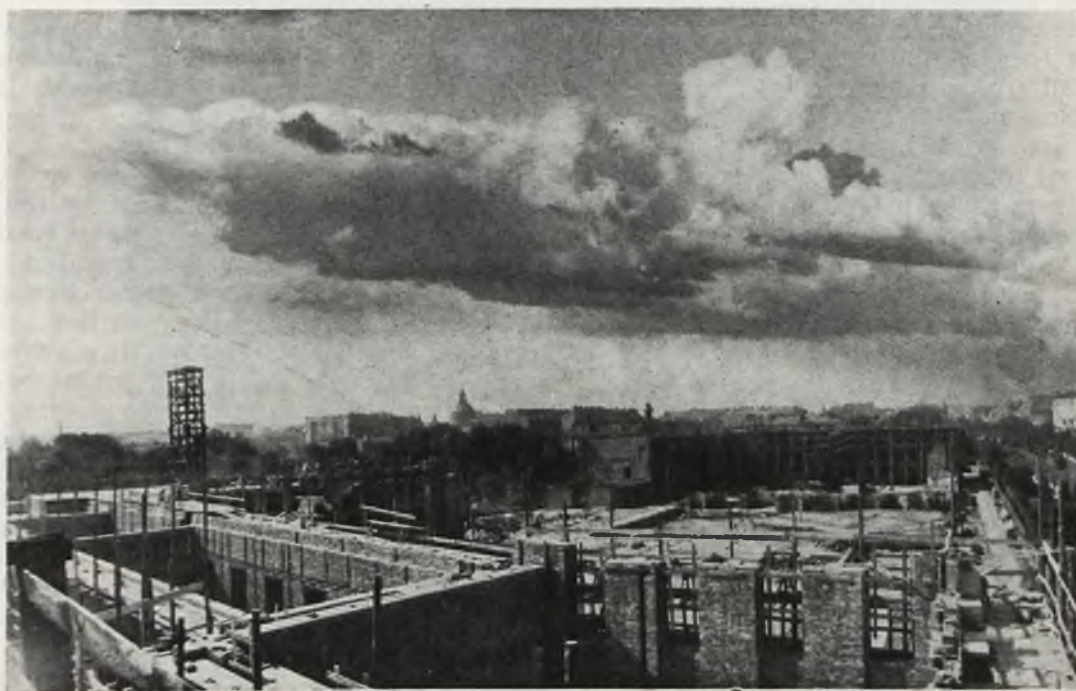
THE CONSTRUCTION OF THE NATIONAL MUSEUM, WARSAW (PHOT. S. PLATER)
