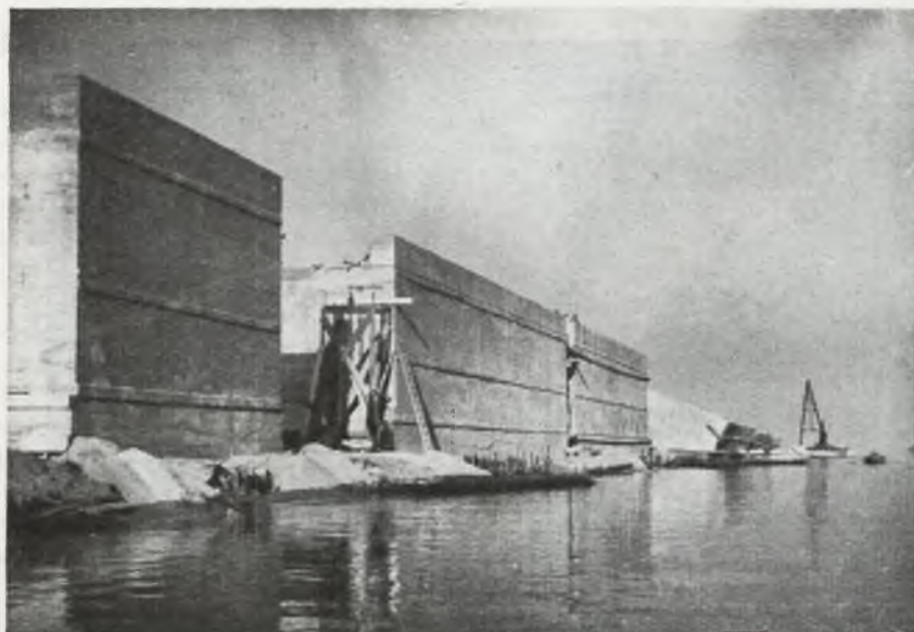
CAISSON SINKING IN GDYNIA (PHOT. S. PLATER)
