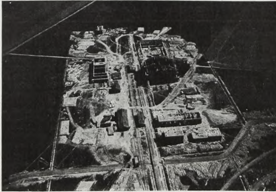
NITRATES FACTORY UNDER CONSTRUCTION AT TARNÓW
