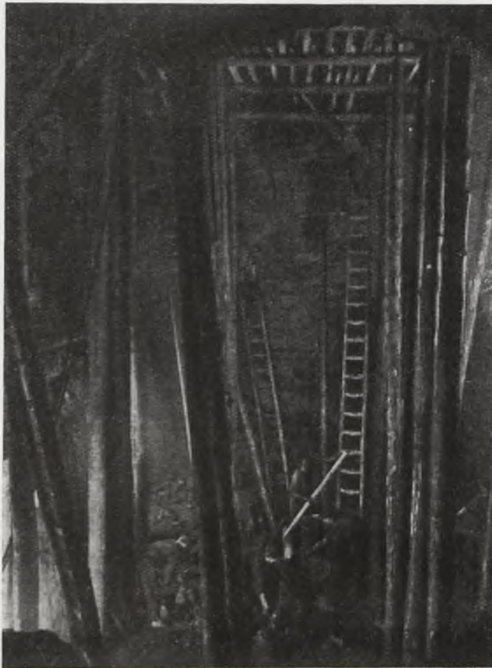
TEN METRE PILLAR IN THE "KRÓL" SHAFT, UPPER SILESIA
