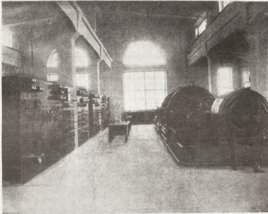
TRANSMITTING ROOM AT THE WIRELESS STATION "RADIO-WARSZAWA"
