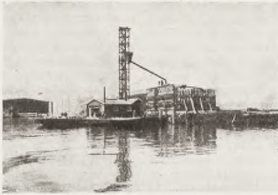
CONSTRUCTION OF CEMENT CAISSONS AT GDYNIA
