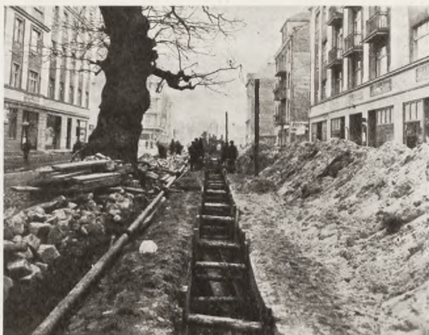
CONSTRUCTION OF A SEWER AT GDYNIA (PHOT. S. PLATER)
