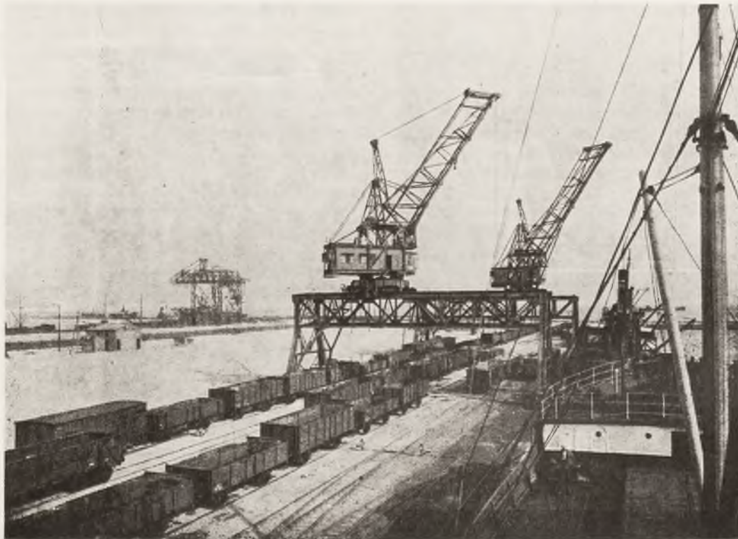
LOADING COAL AT GDYNIA
