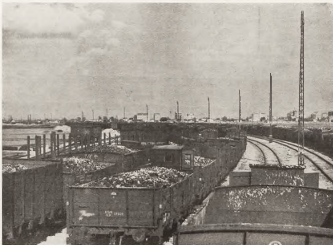
A COMPLETED SECTOR OF THE NEW SILESIA-BALTIC RAILWAY
