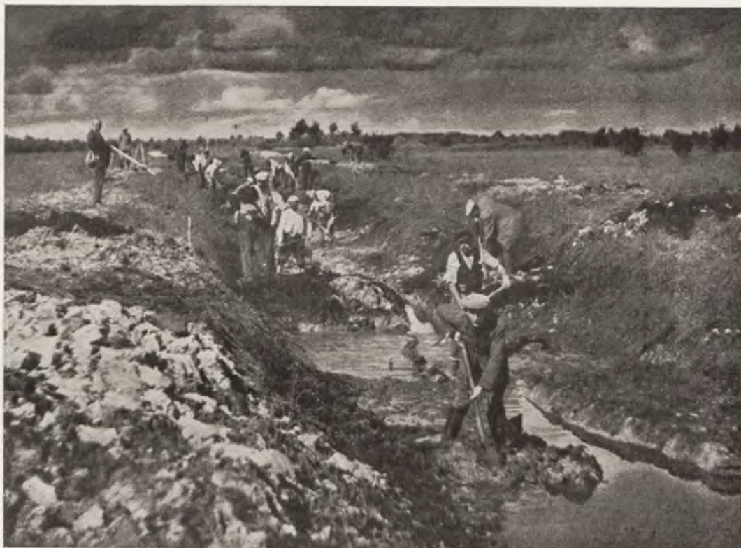
EXCAVATING IRRIGATION CANALS IN EASTERN POLAND
