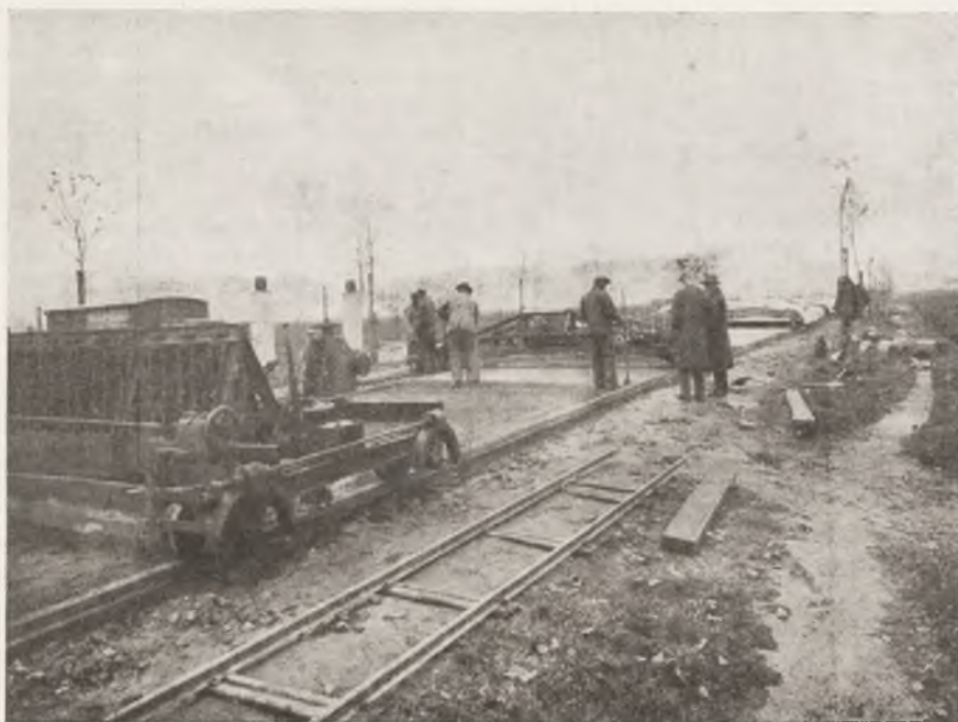
ROAD-CONSTRUCTION IN POLAND
