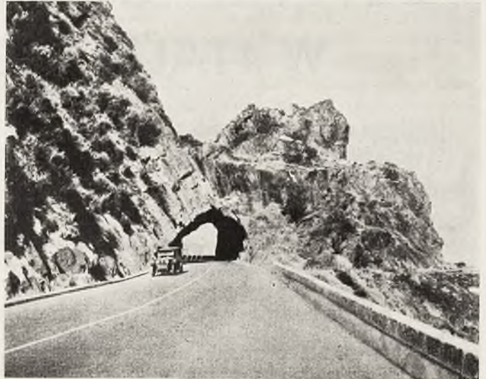
Tunel w Arenzano
