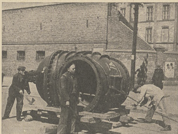
Rys. 1. Transport zasuw D = 1200 mm.
