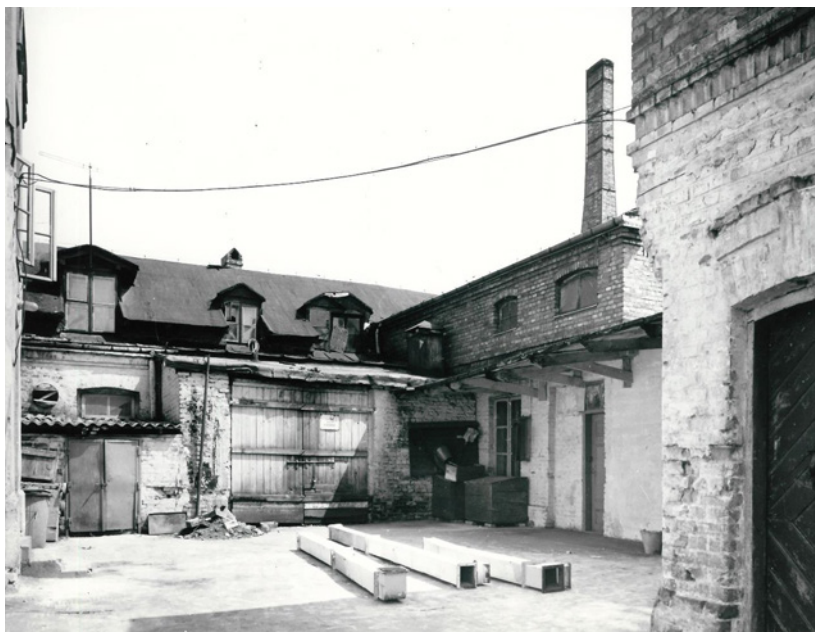
The inner yard, 1976 [from the collection of MWKZ]
