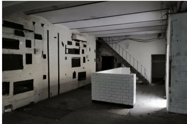
The interior of Piekarnia – view on the stoves [photo by PragaLAB]
