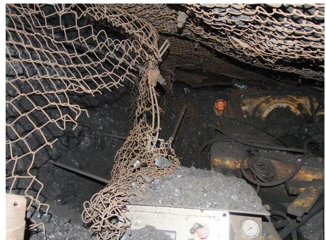
**Fig. 4** Deformation of the roadway caused by a rockburst
