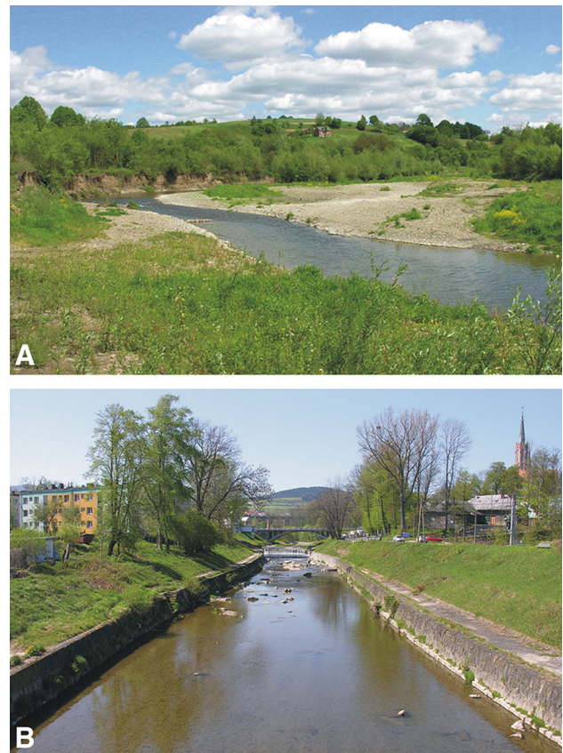
Fig. 2 Examples of near-natural (a) and extremely modified conditions (b) for lateral connectivity of the river ecosystem and channel migration. The unmanaged, sinuous channel can freely migrate on the floodplain. The mode of river channelization presented in the lower photo results not only in the lateral stability of the channel but also in the loss of lateral connectivity of the river ecosystem
