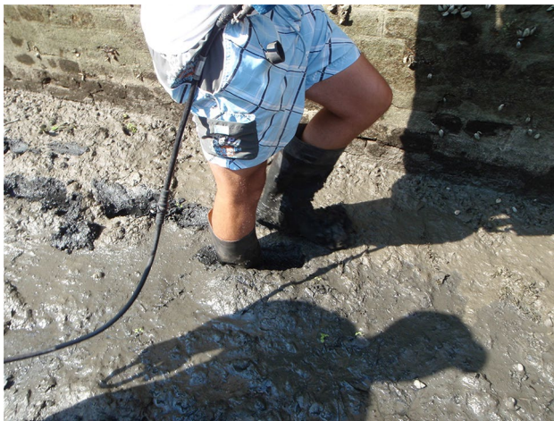
Fig. 4 Bottom of the navigation channel after removing the water
