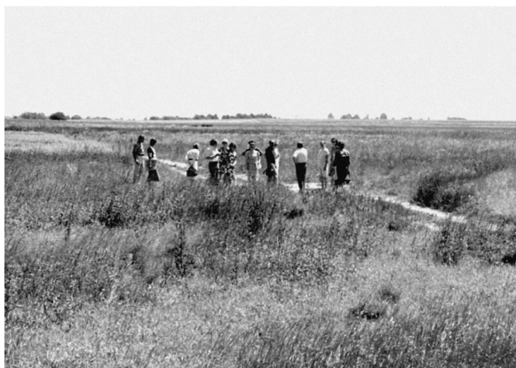
Figure 26. Fields in Ursynów, where the Oncology Centre is to be constructed – a visit of the team of the Surgery Clinic, 1974 (from the collections of the editing office of the MSCNRIO)
