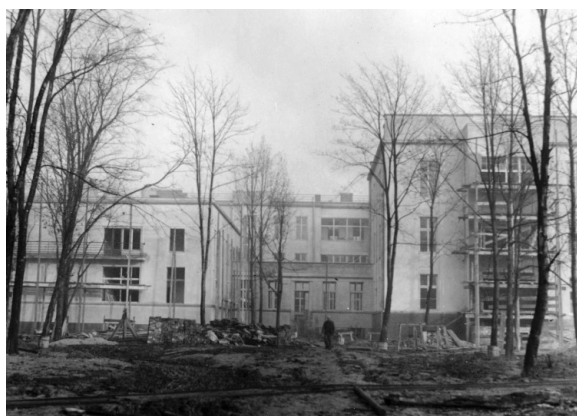
Figure 6. The building of the clinic of the Radium Institute during the completion works, a view from the side of the planned garden (from the collections of the National Digital Archives)
