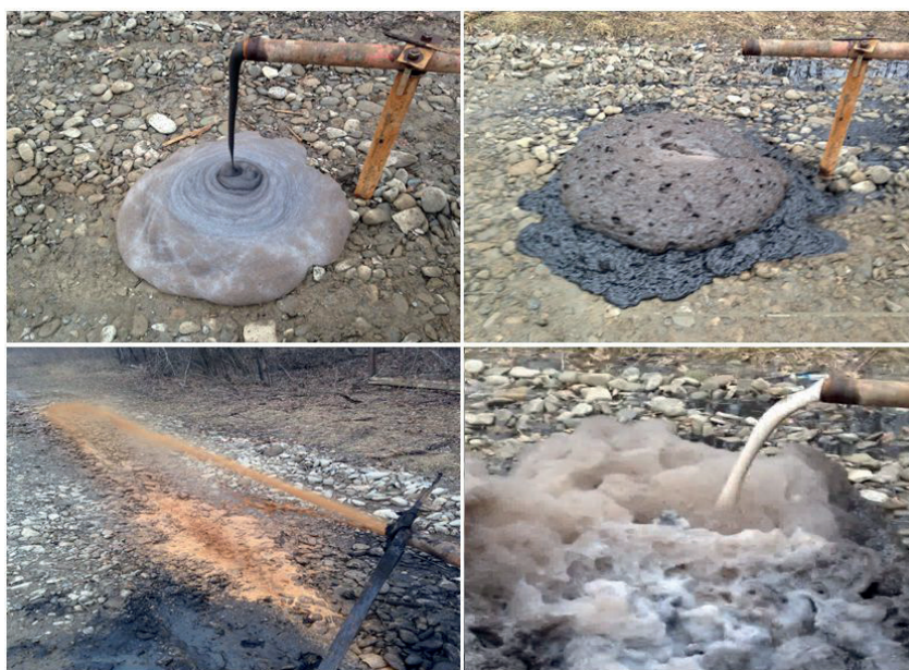
Fig. 15. Removal of colmatents from the well in the form of a gas-foam mixture to the day surface
