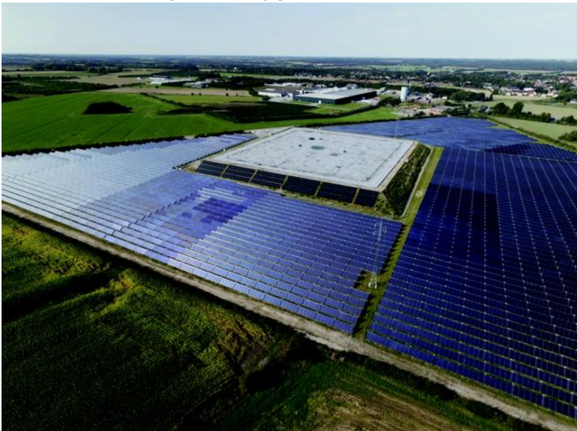
Figure 7. The solar water heating and heat storage pit. (Neimeier, 2021).
