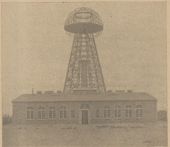
Rys. 4. Budynek Tesli na Long-Island.
