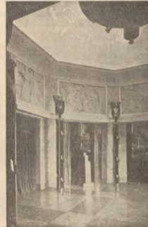
Hall in Polish Pavilion.
