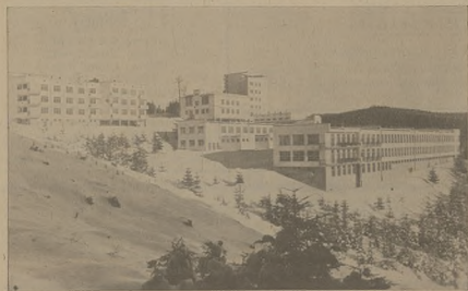
General view of the Sanatorium and School
