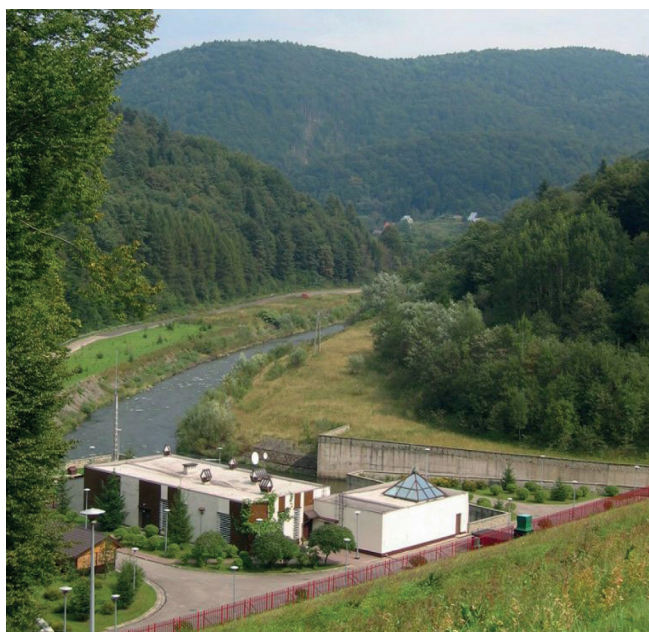
Fig. 6. Hydroelectric power station and the Ropa river valley (Gorlice Pieniny) – view from the dam crest, photo A. Waśkowska
