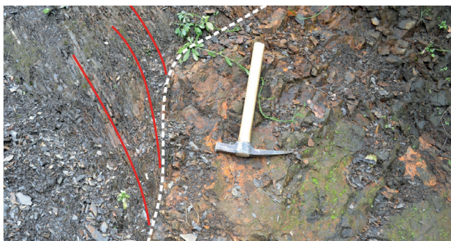
Fig. 5. Contact zone between clastic dyke and shale layers. Bending on the shale layers is underline by red lines (photo J. Barmuta)
