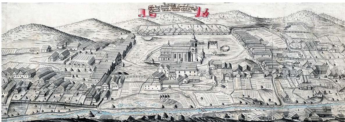
Fig. 30. The mining town of Smolnik in 1748, Slovak mining archive B. Štiavnica
