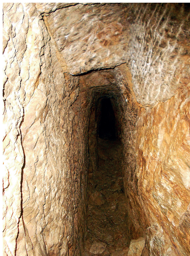
Fig. 22. Manually excavated medieval mining galleries “kresanica“ with a hammer and pick technology in the underground of Lubiětová (Podlipa), photo P. Hronček
