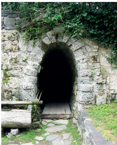
Fig. 43. The “Denná gallery” at Špania dolina, near Banská Bystrica, where Princes Leopold II and Jozef II stepped in to the underground in July 1764, photo P. Hronček
