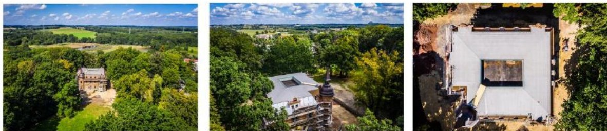
Photo 3-5. Panoramic views of the palace, the roof containing a hidden terrace in the middle and the flat part intended for the photovoltaic panels, 2020 (Author: M. Giba)
