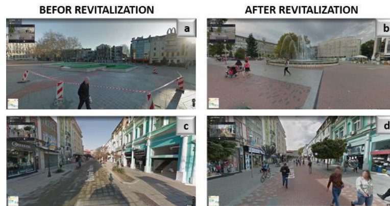
Fig. 10. Modernization of Varna city center (Street View): view of Fountain on Nezavisimost Square (2012 – a), (2019 – b); view of "Kniaz Boris I" Blvd. (2012 – c), (2019 – d)
