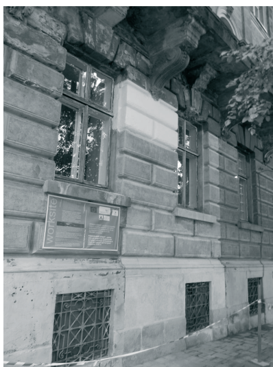
Fig. 4. The fragment of elevation of former “Palace of Justice” after the cleaning, made under promotion prof. J.Weber during the workshop in Lviv as the cooperation between the EU-FP7 project N226898 ROCARE. Aim was to demonstrate the possibility to recover the genuine appearance of the historic elevation by the use of Roman cement as historically authentic and compatible material. Executors were: Atelier Gurtner Wien (Austria) in cooperation with the restoration team of Department of Restoration of architectural Complexes of L'viv Polytechnic. August, 2011.
