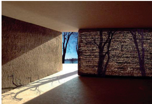
Fig. 7. Synergism in participation: architect as a materials scientist. To the left: residential house with envelopes made of glass-fiber reinforced material; designed by A. Burov – a co-inventor of glass-fiber reinforced material, 1956, Source: http://famous.totalarch.com/burov . To the right: main entrance door of Museum Cella Septichora made of 10cm thick Litracon Classic blocks, 2006, Pécs, Hungary; Bachmann Architects (right). Source: https://www.flickr.com/photos/eager/15739911236 .
