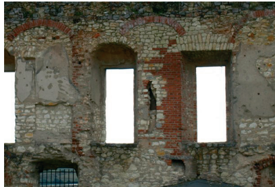
Photo 8. Fragments of the wall rebuilt /castle in Janowiec/
