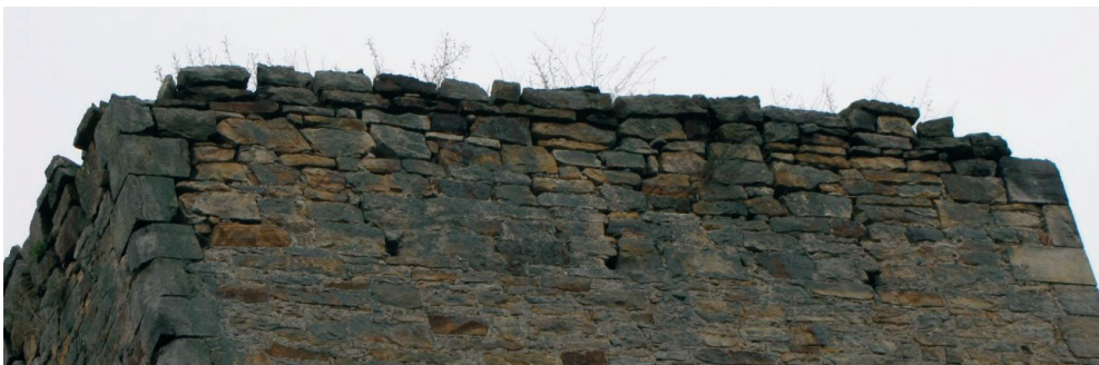
Fig. 12. Degradation of the crest of a stone wall constructed of a really durable material caused by the effect of rainfall and snowfall.
