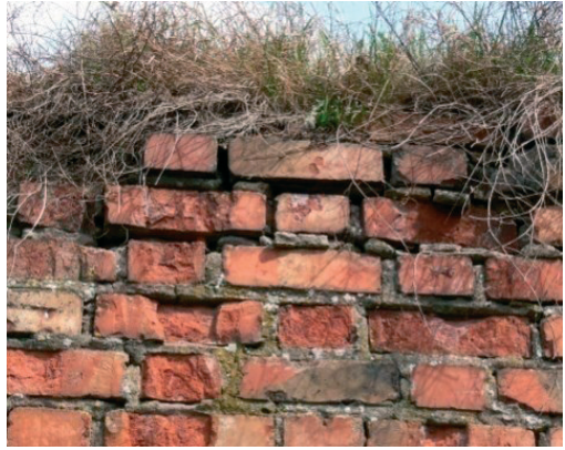
Fig. 15. Degradation of the wall mortar with a good preservation of the wall material.
