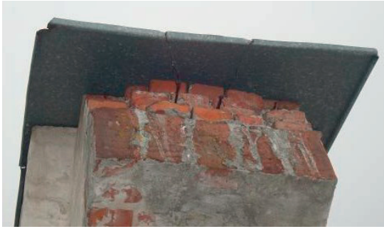
Fig. 32. A steel sheet roofing of the wall crest made directly upon the wall (The castle in Janowiec on the Vistula River)
