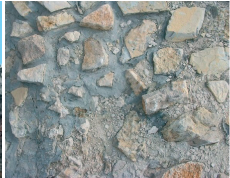
Fig. 37. The degraded chemical cover of the crest.(The castle in Rabsztyn)
