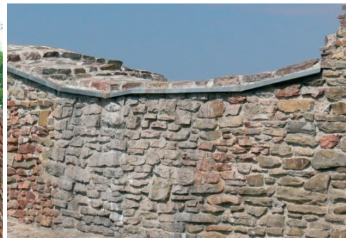
Fig. 23. Addition of the material compatible with the historical one combined with the isolation of sheet metal
