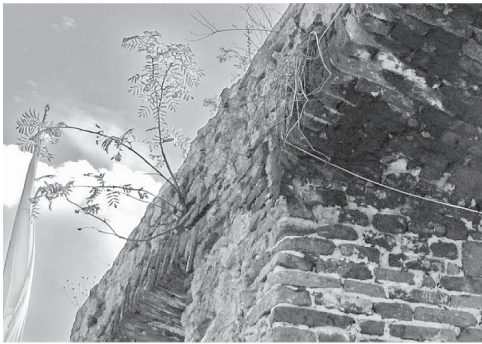
Fig. 15. The rowan rooted in the gap between the wall of the crown and the lintel
