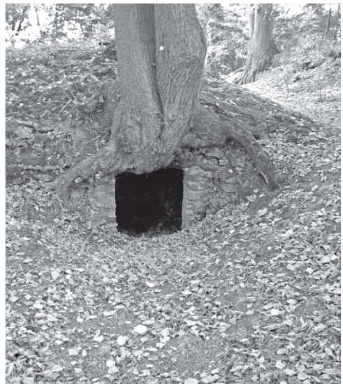
Fig. 18. A huge tree and its root system, which overgrown a stone vault
