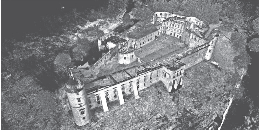
Fig. 3. The cloud of points, which was created as a result of the preparation of spatial data obtained from the Leica C10 scanner – the Janowiec castle
