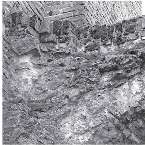
Fig. 6. Moss and algae, which overgrow the crown and the face of the wall
