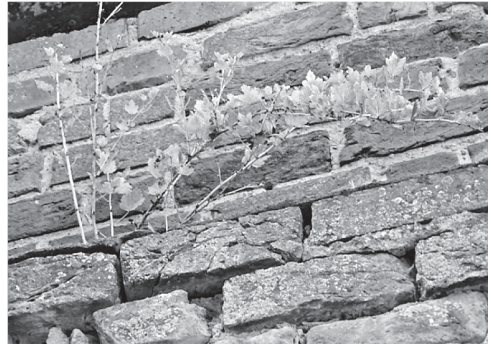
Fig. 16. A shrub with a root system overgrowing a ceramic brick wall
