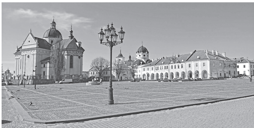
Fig. 3. Today photo of central square of town of Zhovkva, M. Bevez, 2018
