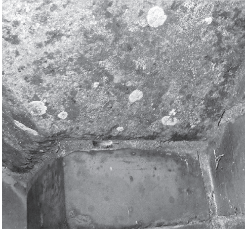
Fig. 3. A fragment of the plastered ceiling overgrown with lichens
