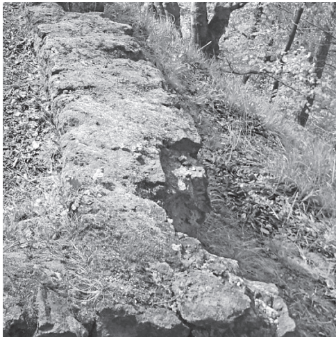
Fig. 5. Mosses growing on the low crown of the north wall of the ruin
