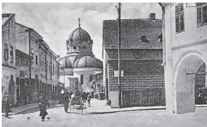
Fig. 18. The corner of building loggias-arcades from the side of Korotka street (Skorzana street in the past) on the post card of 1909. [50]. Basilian monastery is on the second plan
