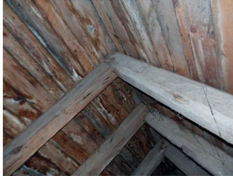
Fig. 13. Nowa Kościelnica – connection of the rafter (author's own photography)
