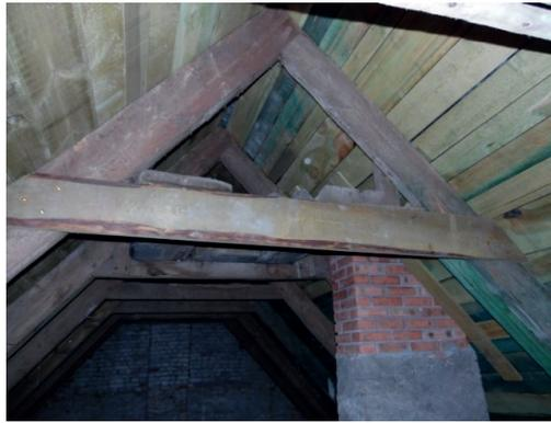
Fig. 17. Rybina – a new collar beam in the structure (author's own photography)
