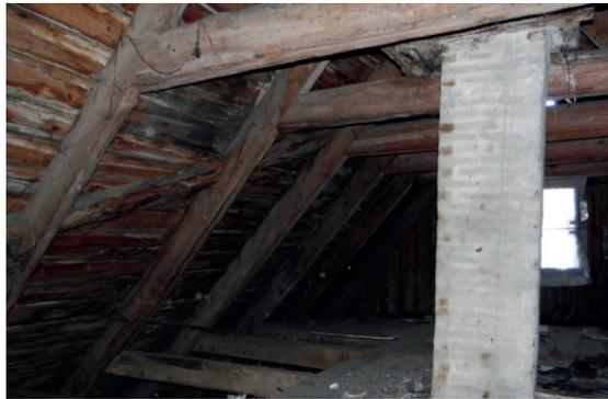
Fig. 10. Marynowy – the view on the rafter framing with two collar beams (author's own photography)
