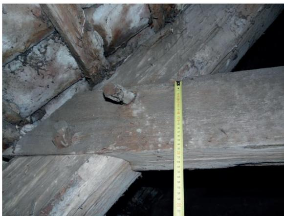
Fig. 8. Bystrze – connection of a collar beam with a rafter. (author's own photography)
