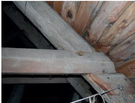
Fig. 14. Nowa Kościelnica – connection of the rafter with the collar beam (author's own photo.)
