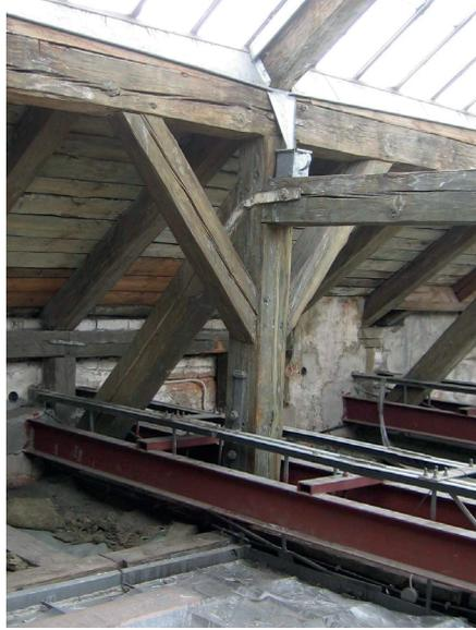
Fig. 4. Steel load bearing elements taking over the bearing role of original wooden elements (photo. A. Halicka)
