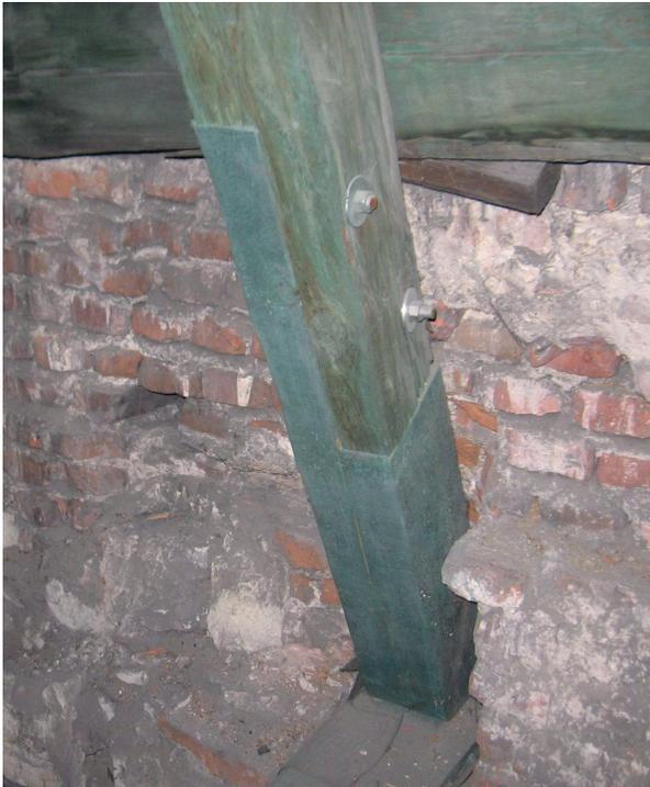
Fig. 2. Replacement of the rafter support zone with a new wooden part (photo. A. Halicka)
