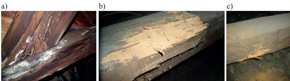
Fig. 1. Damage to wooden elements: a) structural elements affected by fungi (photo. Sz. Ślósarz); b), c) structural elements destroyed by insects, (photo. Sz. Ślósarz, A. Halicka)
