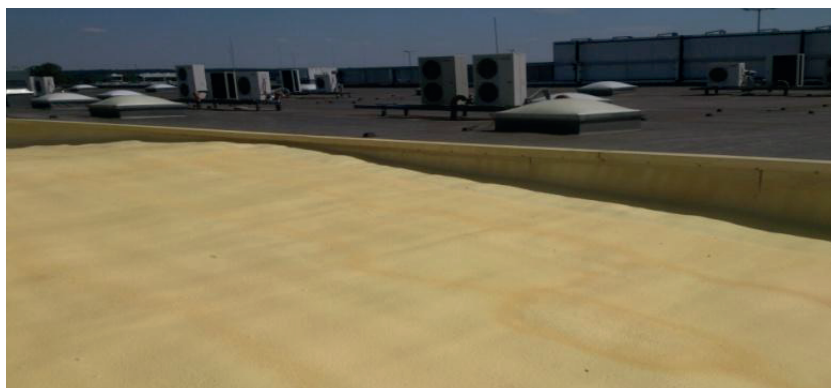
Fig. 2. The roof after the restoration with the use of the plastic foil. Higher level of aesthetics. Source: R. Pilch
