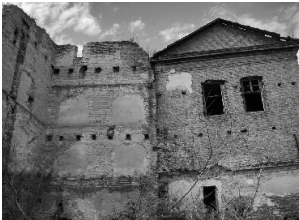
Fig. 4. Klevan Castle. Current status. View of the inside of the west tower. Photos by N. Leshchenko
