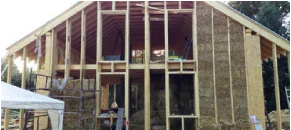
Fig. 1. Implementation of the ‘straw house’ project 2014/2016, Koziej Architekci office (source [14])
