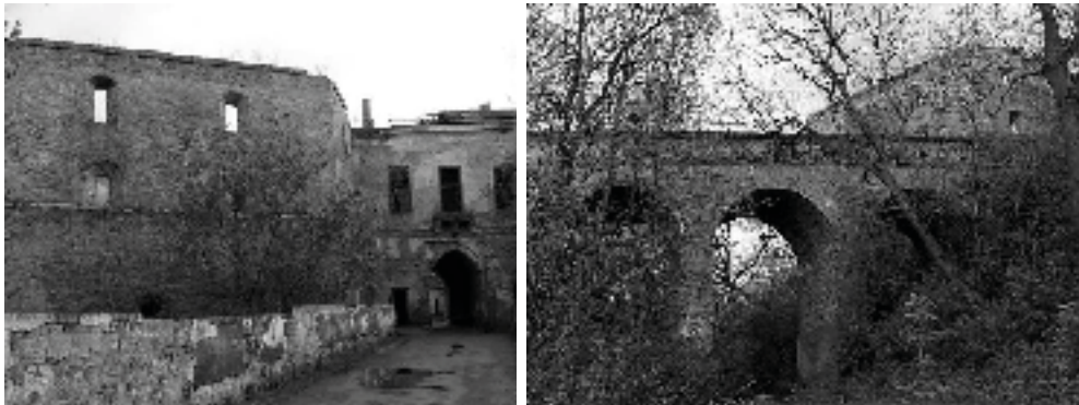
Fig. 2. Klevan Castle. Current status. View from the entry bridge. Photos by N. Leshchenko
