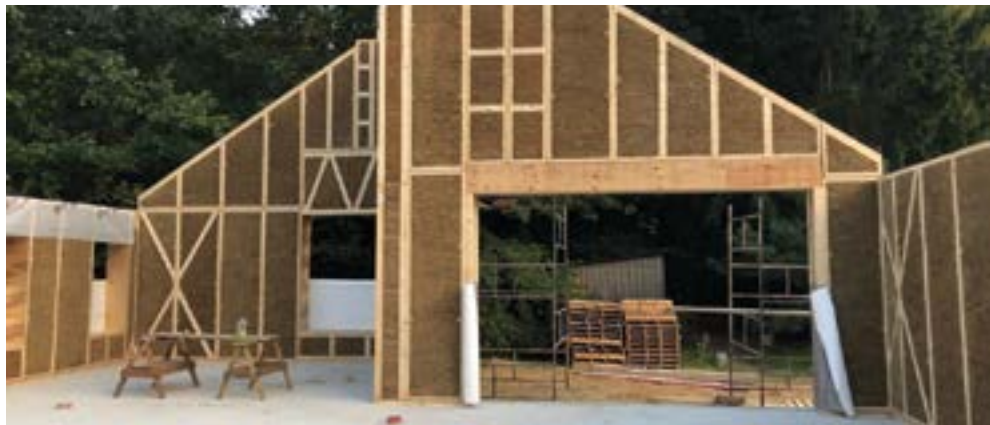
Fig. 2. Implementation of the ‘ASZ Dom’ project using prefabricated EcoCocon panels, Koziej Architekci office, source: www.koziejarchitekci.com [14]
