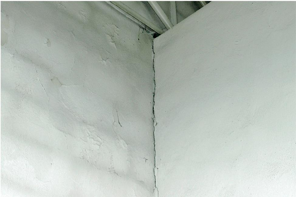
Fig. 11. Cracks at the junction of the masonry partition wall of the second storey with the western gable wall.
