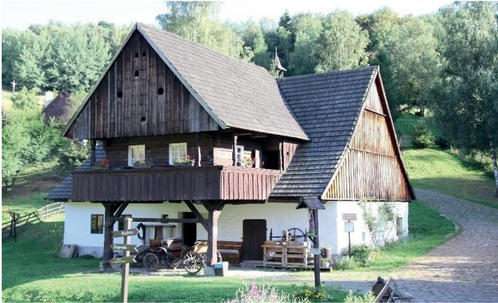
Fig. 3. Pstrązna – an open-air museum of wooden buildings. The so-called *Zajazd* (Inn) moved from Szalejów Dolny (probably built in the first half of the nineteenth century). The modest form of a single-storey house with log walls is diversified by an attic storeroom, i.e. an extension protruding beyond the eaves, supported on posts, in which there were rooms for tourists. *Photo by Jacek Suchodolski 2015*
