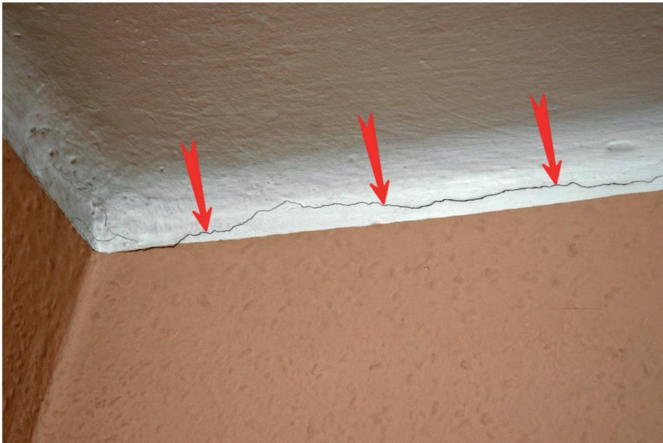
Fig. 6. Gap of up to 1.5 mm between ceiling and first floor interior wall. *Source: author*
