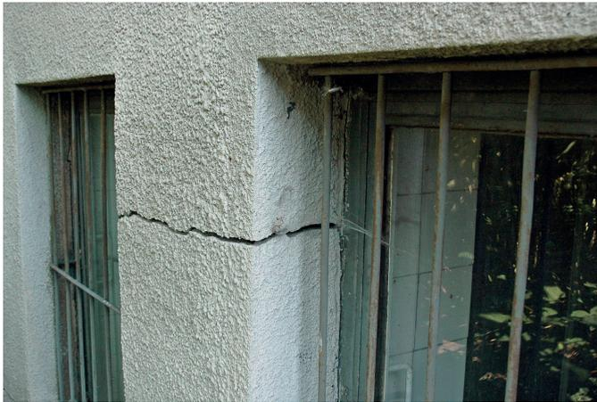
Fig. 9. Fragment of the basement wall of segment 1 – visible cracks in the inter-window pillar from the outside and no damage at this point inside. *Source: author*
