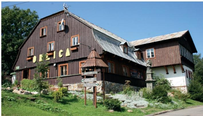
Fig. 4. Orlica shelter in Zieleniec, built in 1878. The building with log walls, covered from the outside with vertically-laid boards and with a mansard roof with dormers, also has an attic storeroom in the form of an extension, supported by the masonry walls of the ground floor. There was a second tavern near Orlica (*Gasthaus zur Mense*), of a similar shape and structure, but it was pulled down in the 1960s. *Photo by Jacek Suchodolski 2009*
