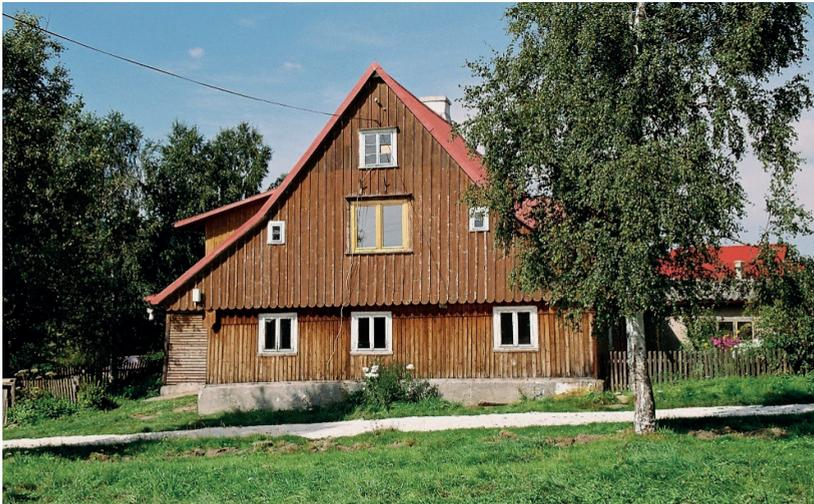
Fig. 13. Lasówka (*Kaiserswalde*). Former *Erlitztalbaude* shelter, now a residential building. The metal sheet on the roof was nailed to the original shingle covering through ridge beams. Photo by Jacek Suchodolski 2005
