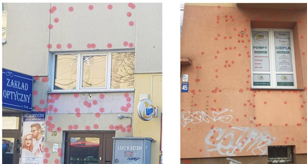
Fig. 9. The points highlighted in red are holes left after repeated removal of advertising signs, *Source:* Author
