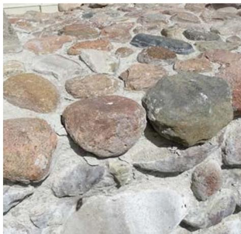
Fig. 16. South-east wall. Damage to joints, detachment of individual tones of face and top layers. *Source:* author, 2019
