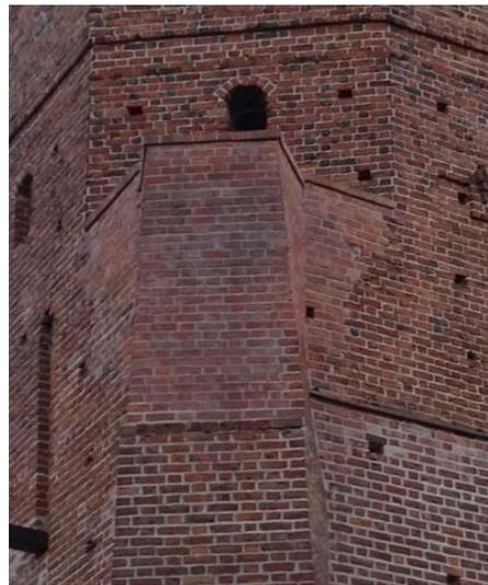
Fig. 14. Tower, view of south-west elevation. The repointed wall topping of the tower buttresses. The brickwork and pointing used ensures that the layers are distinguishable. *Source:* author, 2019
