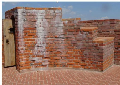
Fig. 6. Tower wall topping. Severe salt corrosion of the brick face of the tower terrace exit. Salt corrosion damaged brick faces. Carbonate streaks on the surface of the masonry. *Source:* author, 2019
