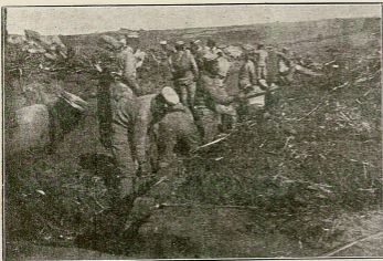
OUR ENTRENCHING WORK NEAR THE SHA-HO
