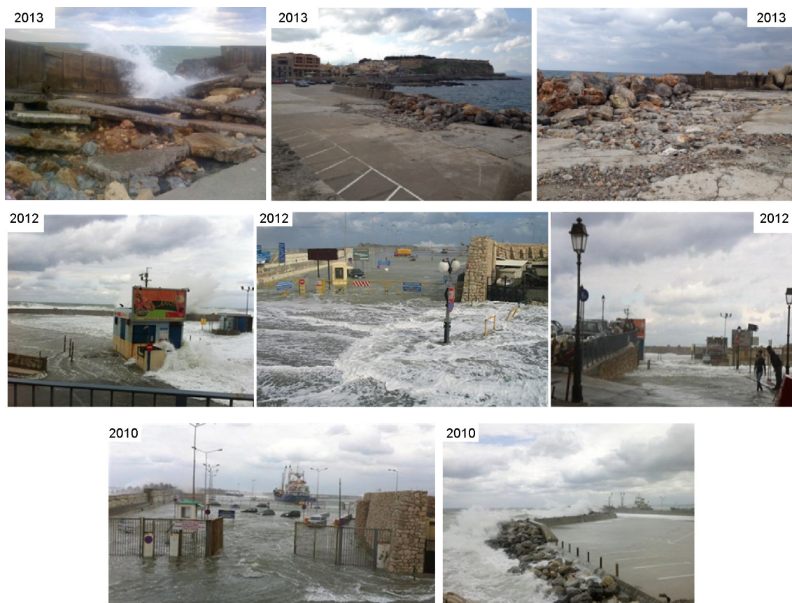
Figure 3 Recent floods at the harbour area of Rethymno (2010–2013).
