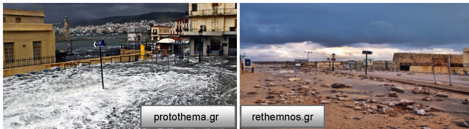
Figure 5 Penetration of seawater through overtopping to the wider area of port facilities and debris from the windward wave breakwater damages.
