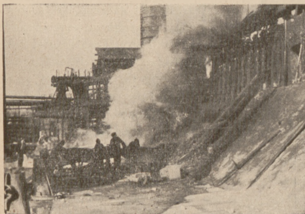
Part View of the Coke-oven Plant at „Zabrze“
