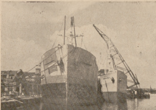
Ship Repairs in Gdańsk Shipyard.
